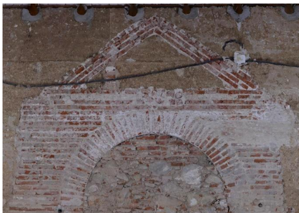
Figure 14. Detail of the front and the semicircular arch of the new open portal on facing 2
