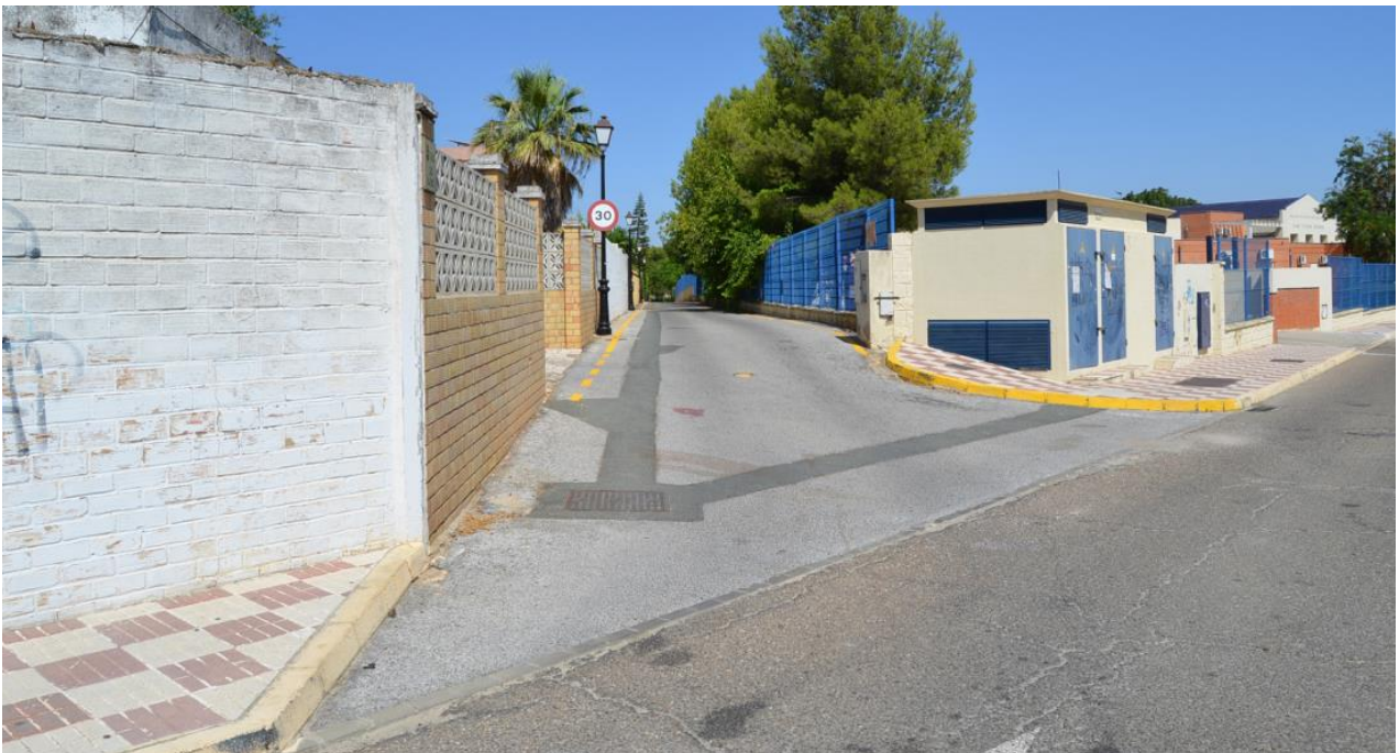
Figure 7. Access road to Los Álamos, municipality of Bormujos. The authors (2023).
