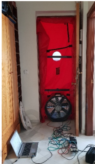
Fig. 2. Blower Door test development in Case 4 dwelling. The photograph is taken from the inside.
