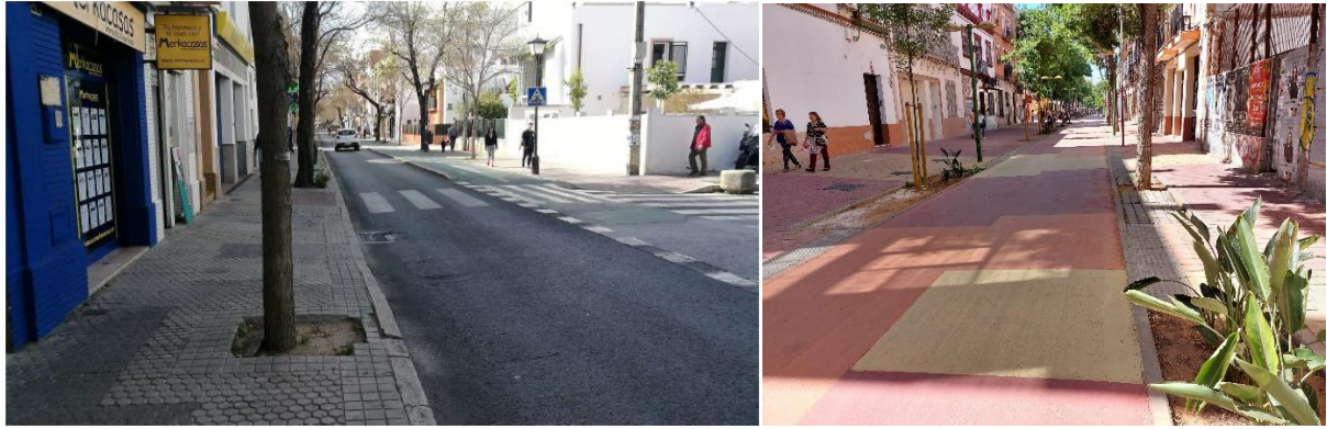
Figure 13 – Street before (left) and after (right) rehabilitation works
