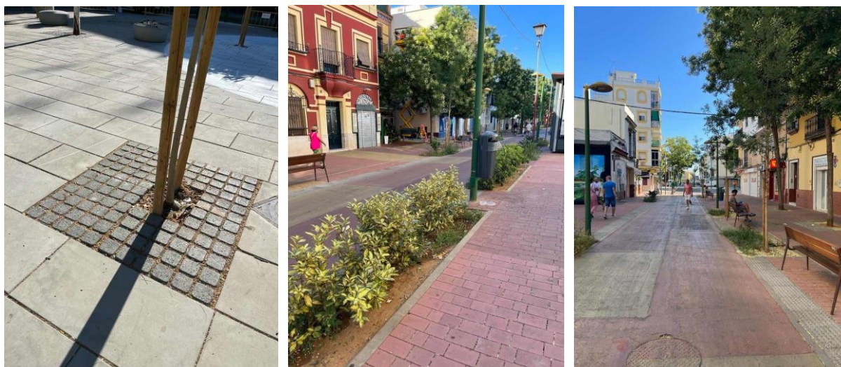
Figure 25 – Pictures of the section after rehabilitation works
