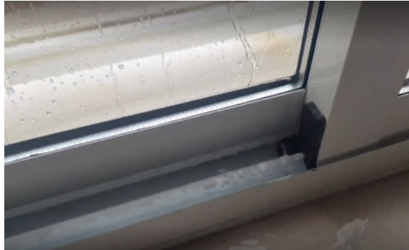
Fig. 7 Window during test
