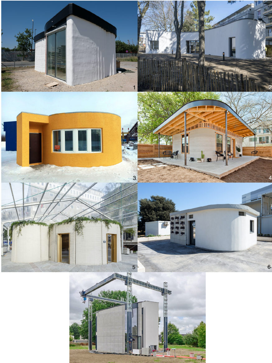
Imagen 2. Ejemplos de Viviendas Impresas (fuentes: https://cobod.com/the-bod/ ; https://theculturetrip.com/europe/france/articles/the-first-3d-printed-home-in-the-world-has-been-unveiled-in-france/ ; https://www.businessinsider.com/house-built-one-day-apis-cor-2017-3 ; https://www.archdaily.com/919667/could-3d-printing-be-the-future-of-social-housing ; https://bemore3d.com/language/en/3d-housing/ ; https://theurbandevolver.com/articles/portable-robot-prints-house-in-48-hours ; https://www.kampc.be/innovatie/projecten/3d-printen-in-de-bouw/presentaties-fotos , 2017-2020).
