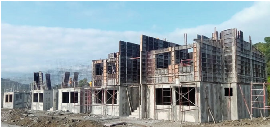
Fig. 9.3 Block of flats under construction, reinforced concrete walls
