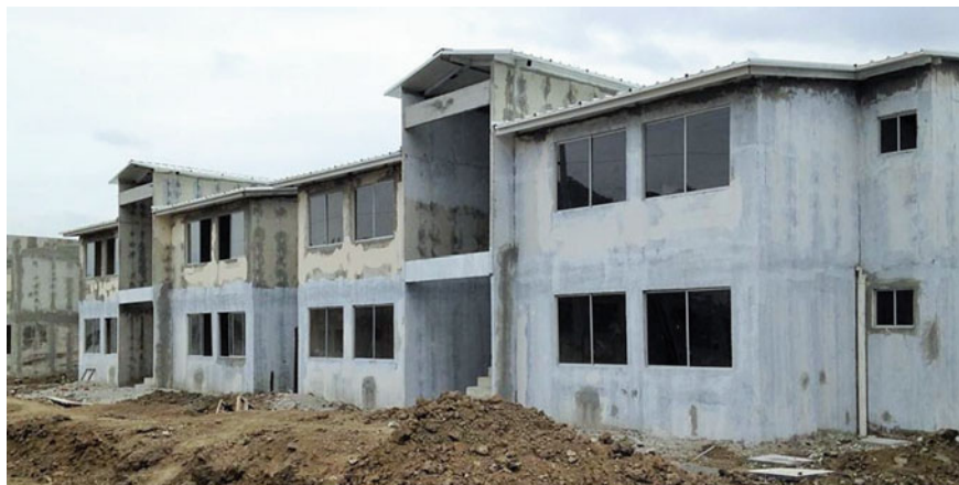
Fig. 9.4 Plastering building, carpentry installed
