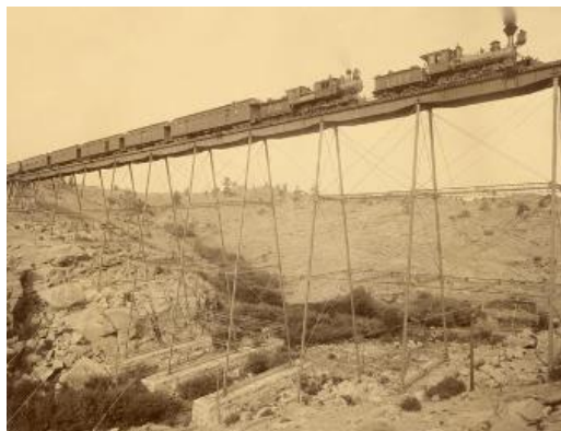
Figura 1. Dale Creek Bridge (Laramie, EEUU) [25]
