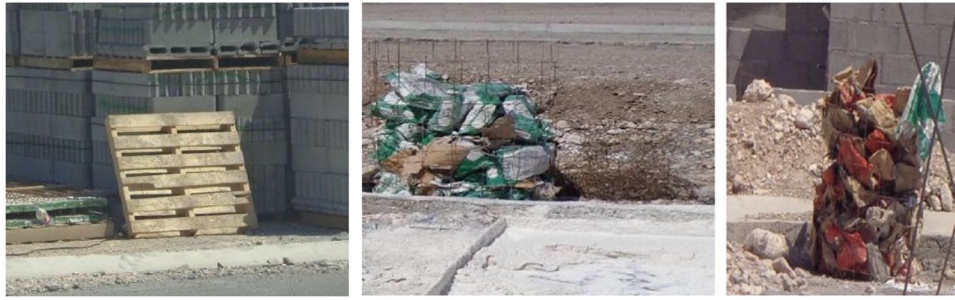
Figure 3. CDW packages stored in the construction site.
