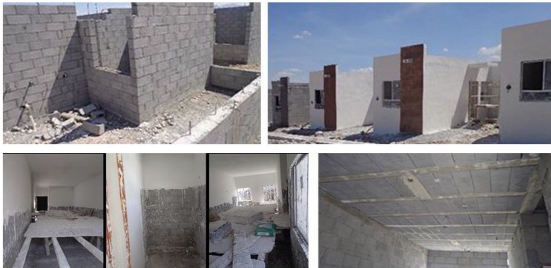
Figure 2. Social housing under construction.
