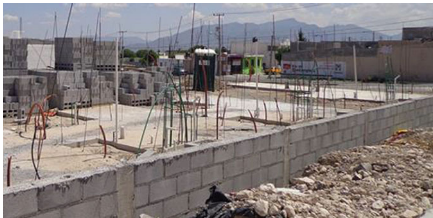
Fig. 4 Social housing under construction. Source The authors
