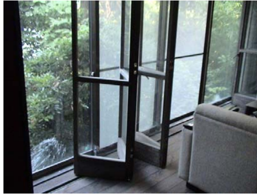
Figure 3. Detail of the pliable window designed by Taut in the Hyûga House at Atami (Japan)
