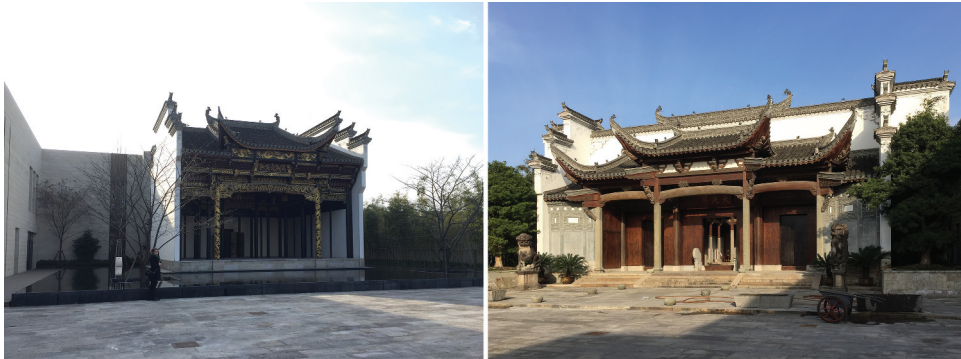
Figure 2. Theatre stage (left) and Ancestral Hall (right) in the entrance courtyard of Ahn Luh Zhujiyajiao. Source: Plácido González Martínez.
