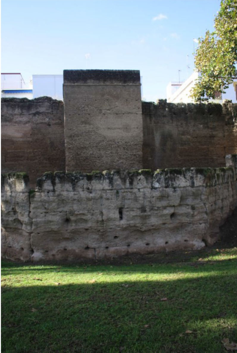
Figure 8. Seville ramparts could be affected by the earthquakes.
