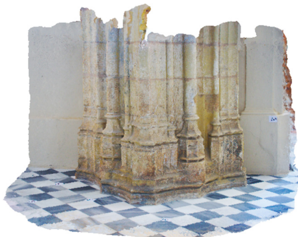
Figure 4. Three-dimensional digital model from the photogrammetry of the pillar of the church in Morón de la Frontera, Spain.
