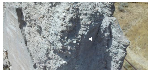
Figure 21. Mark of the headboard of rammed-earth wall 21. Photography: Félix Pérez Moreno 2019.
