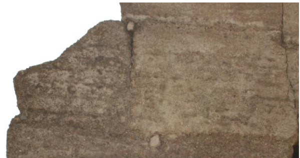
Figure 20. View the putlog holes filled with stones. Photography: Jorge Moya Muñoz 2019.
