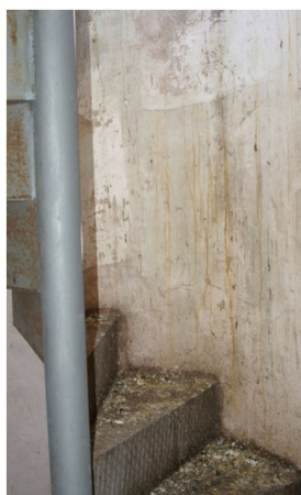
Figure 11. Stairs access to the bell tower.
