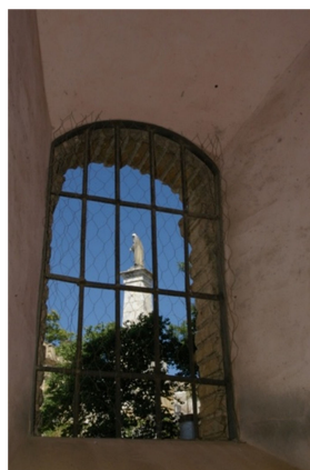
Figure 10. Detail of the current enclosure of one of the windows.
