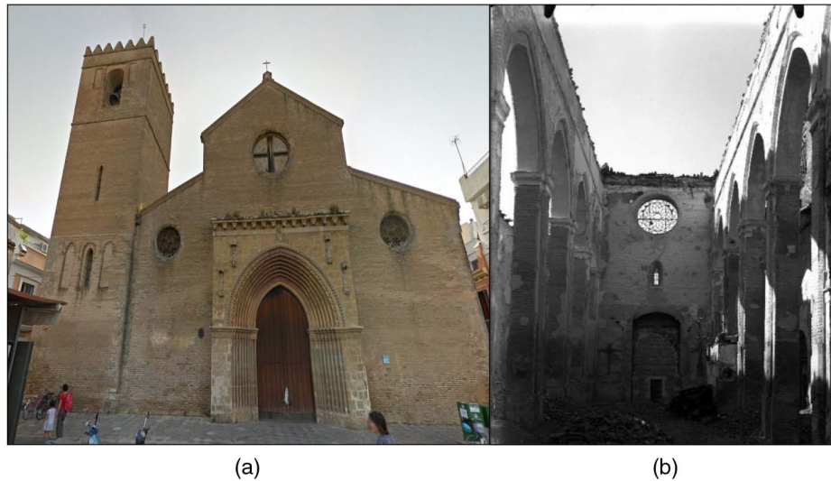
Fig. 8. Illustrative case studies in the serviceability range conditions: (a) Santa Marina church in 2016 (Seville) (image by A. J. Prieto); (b) Ominum Sanctorum church (Seville) (image courtesy of the University of Seville)
