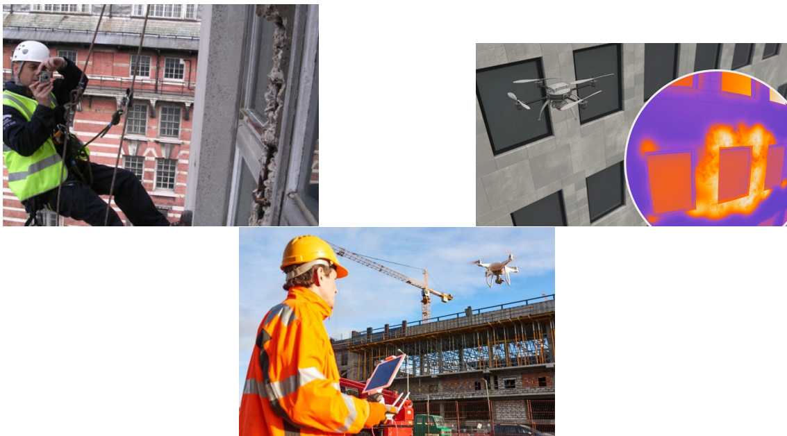
Figure 1.1 Worker and drone in building inspection.
