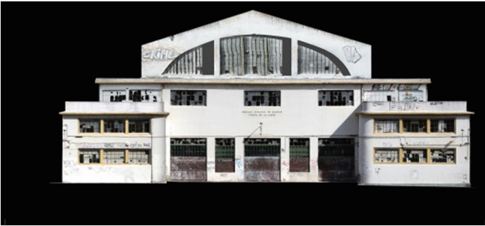
Fig. 10. Final photogrammetric capture. Orthophoto of the main façade. Author: Roque Angulo Fornos (2015).
