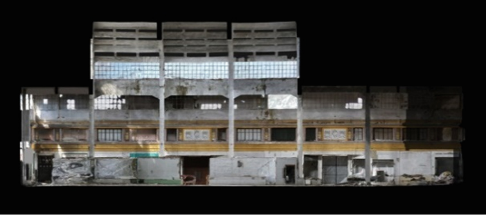
Fig. 9. Final photogrammetric capture. Orthophoto of the longitudinal section through the central space. Author: Roque Angulo Fornos (2015).
