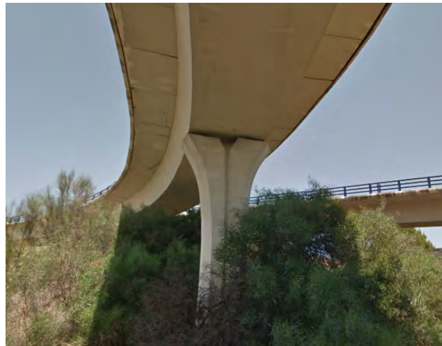
Figure 4.26: Reinforced concrete bridge. Image extracted from Google Maps [1].
