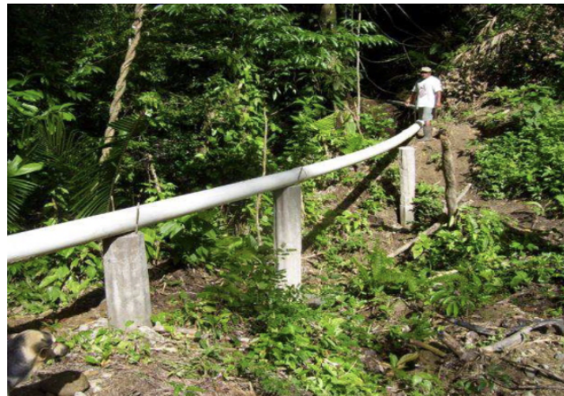
Figure 2. Bending in a real MHPP penstock length.
