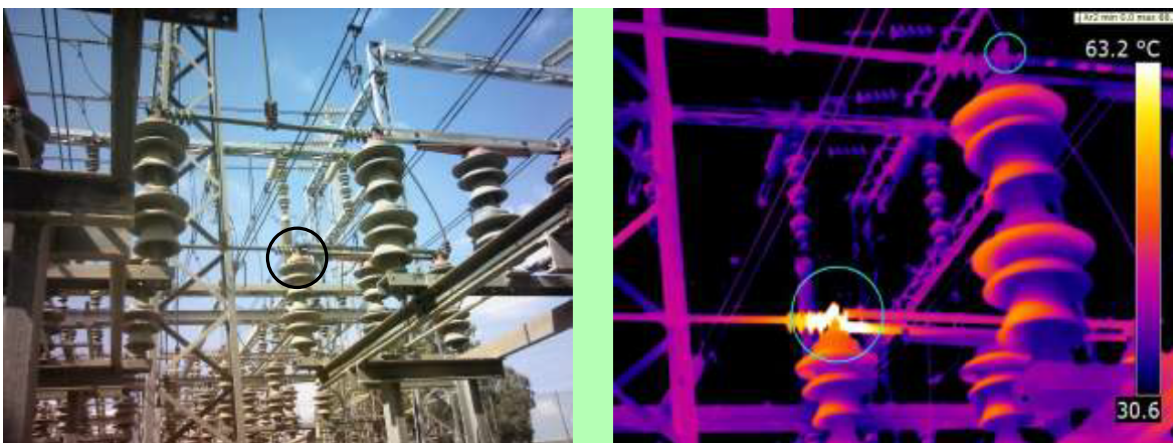
Fig. 1: Normal and thermal images of hot spot: Cu tube with Cu flatbar connector.
