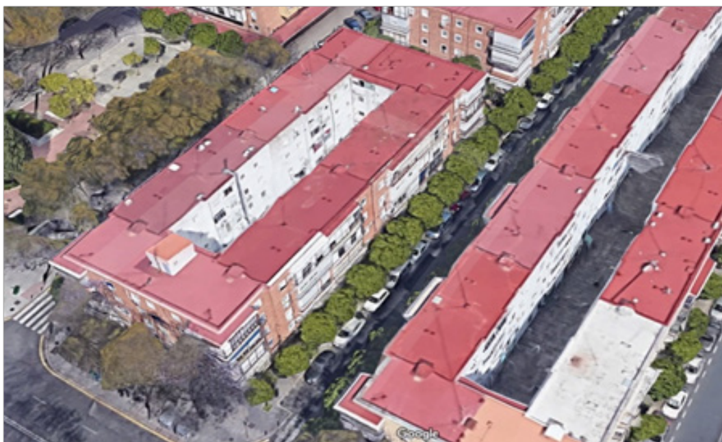
Fig. 1. Buildings from the Juncal neighborhood, Sevilla, (Spain). Source: Own elaboration.
