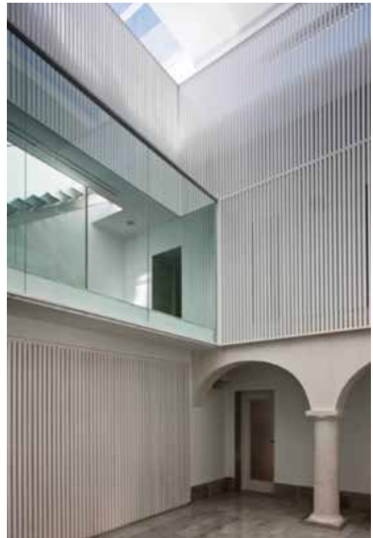
Figure 10. View of the courtyard after the intervention.
