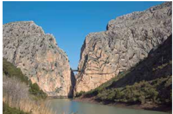
Figure 1. View of the bridge into The Gaitanes Gorge. Author: © Duccio Malagamba, 2015. Source: Luis Machuca y Asociados, S.L.P.
