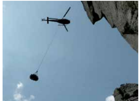
Figure 12. Helicopter delivery of materials and waste management for greater precision and efficiency.
