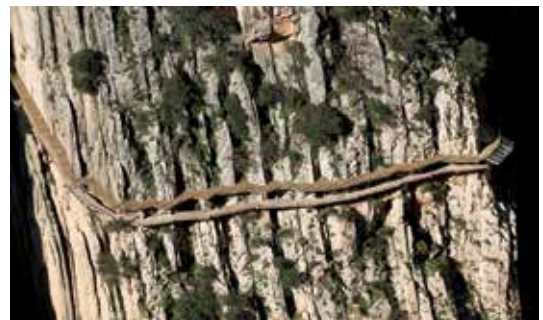
Figure 7. Aerial view of the two footbridges. Author: Juan María. Source: Luis Machuca y Asociados, S.L.P.
