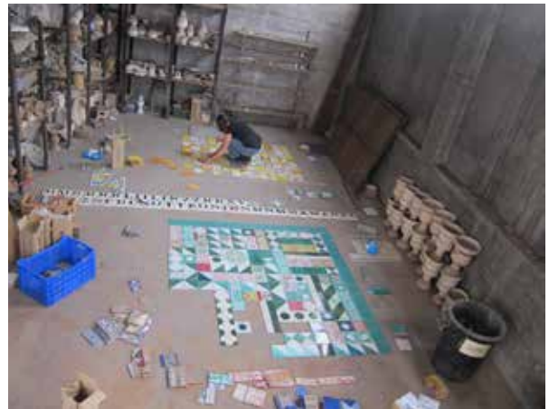
Figure 11. Rehabilitation of the Antigua fábrica de Montalván, Triana, Sevilla (Former Pottery complex Montalván) as Triana Montalván Hotel and Restaurant. Catalogation process of tiles
