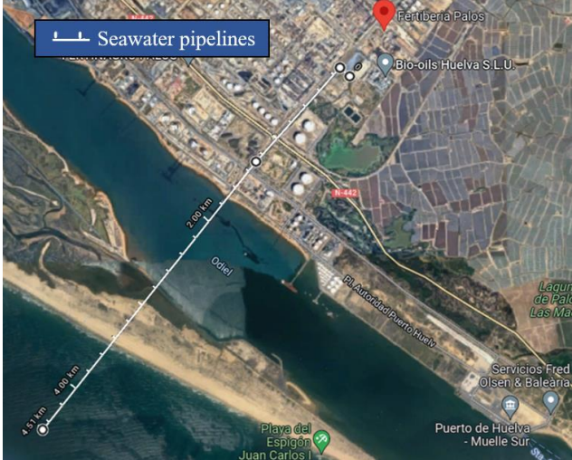
Figure 22. Pipelines crossing Odiel.
