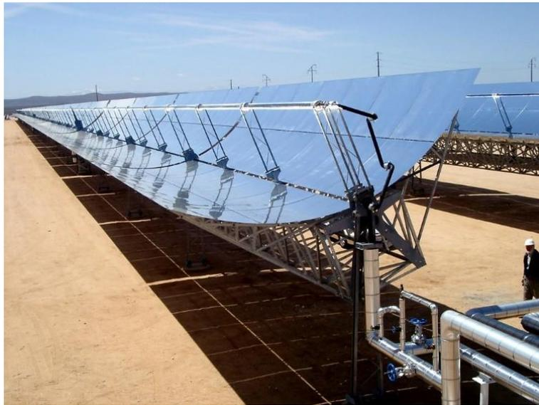
Figura 1-6. Central termosolar CPP
