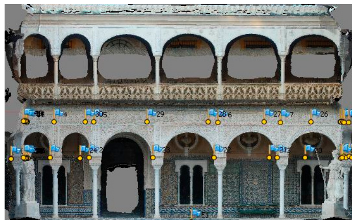
Figure 10. Control point distribution in the northeast arcade.
