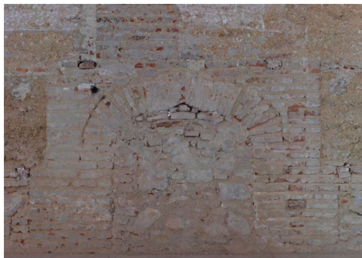
Figure 12. Main door of the original cloister with an ogee arch on the top.
