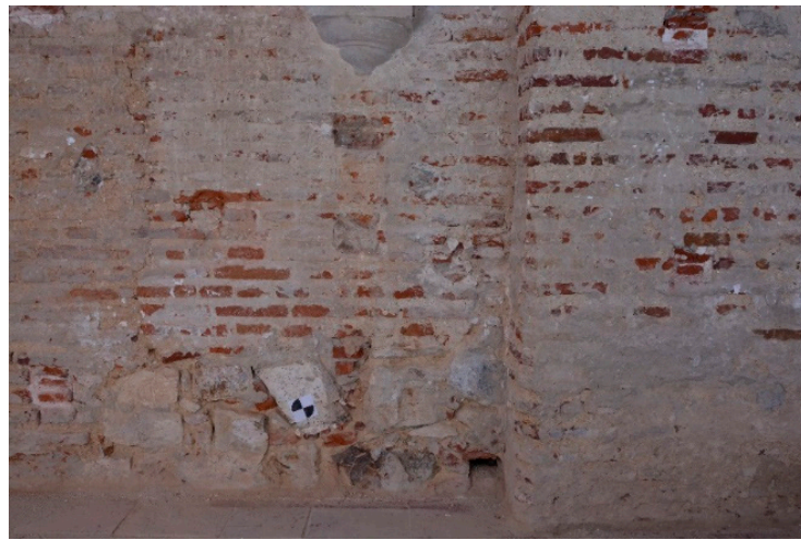
Figure 13. Detailed image of the facing of the church, the original wall and the reforms of the cloister.
