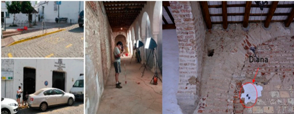
Figure 2. GNSS stationing, placing and measurement of permanent points inside and outside the cloister.
