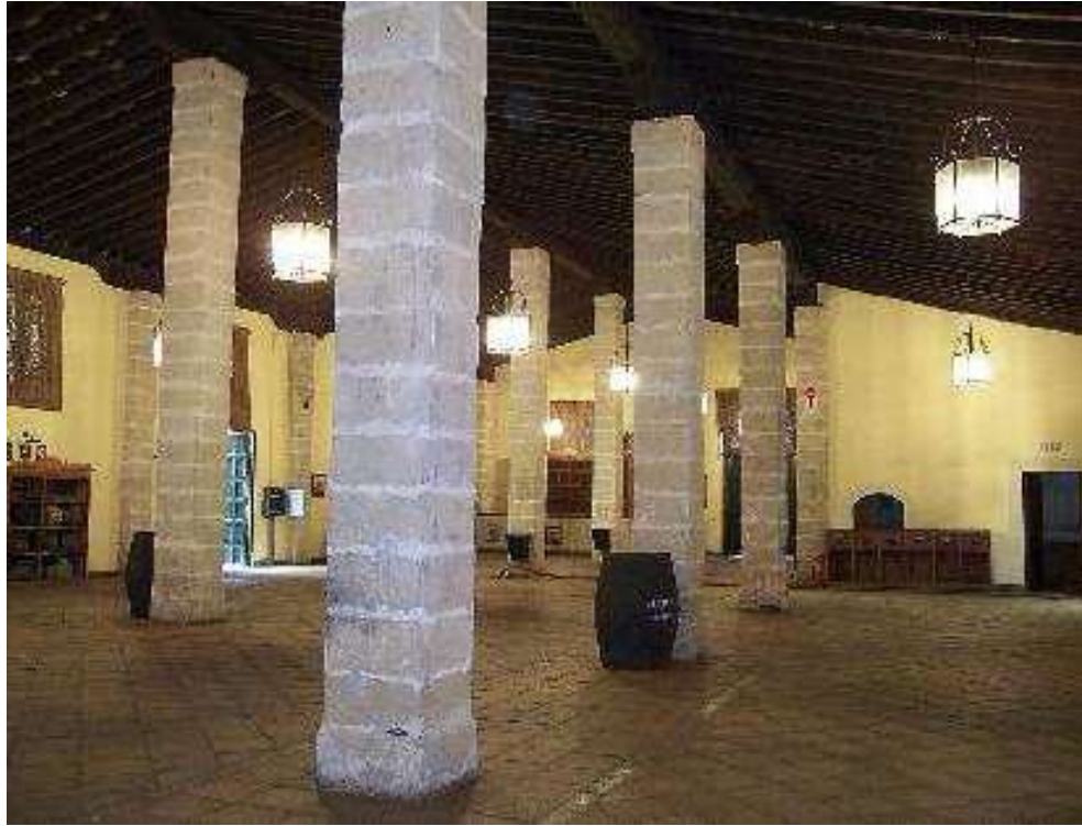
FIG. 4 Emptied at present of his original content, winery (above) and house of vineyard (bellow). They reproduce similar structural and spatial schemes. (Photos of the author and of Jesus Ortúe Vázquez, respectively)
