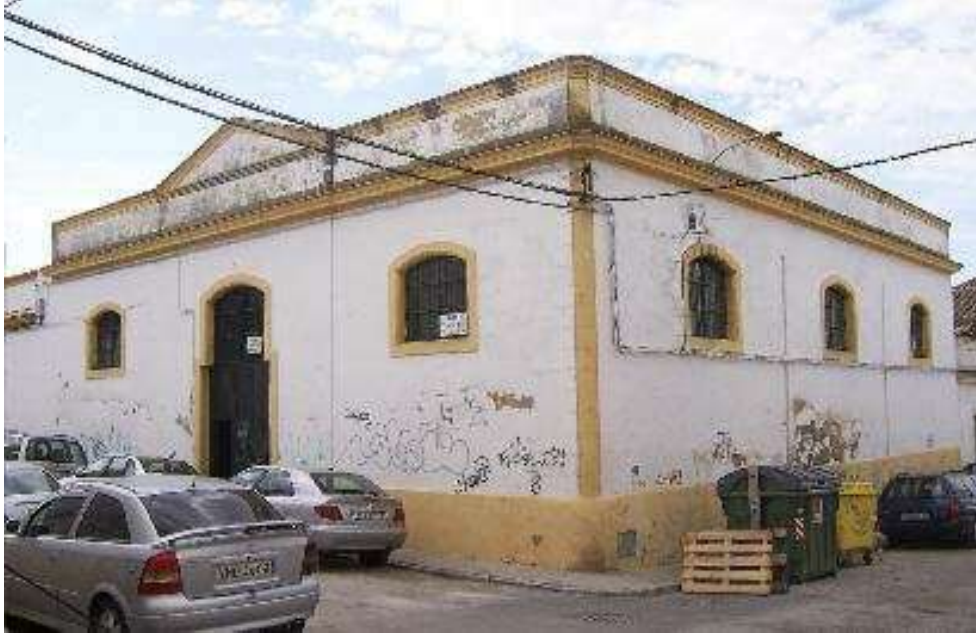
FIG. 3 Front of an urban wine house that conceals the covering (above), and similar solution in the front of the almijar of a house of vineyard (bellow). (Photos of the author and of Jesus Ortúe Vázquez, respectively)
