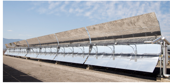
Figure 1: Lateral view of the first TCP-100 PTC in the first loop at Pataforma Solar de Almería (PSA-CIEMAT). It is composed of 8 modules of 12 meters length. Courtesy of PSA.
