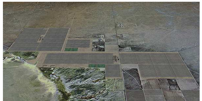
Figura 3: Mojave solar project: Cortesía de Atlantica Sustainable Infrastructure
