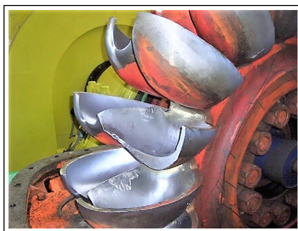
Figure 8. Damage in a bucket.
