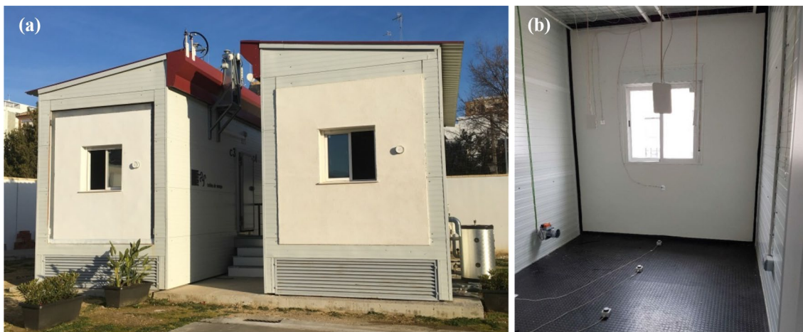
Fig. 2 Test cells located in Seville (southern Spain): a general view; b indoors
