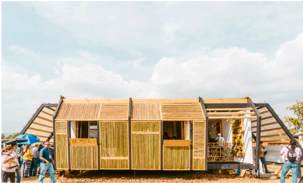
Fig. 1. South elevation of the AURA 1.0 prototype and cane panels as solar protection.
