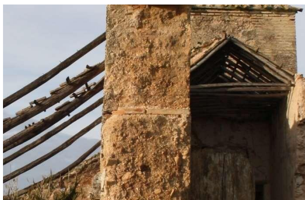
Figure 11: Detail of the rammed earth wall with mortar and a single brick course that separates the different areas at the Gallego mill in Écija. It clearly shows the thickness as two stretcher bricks.
