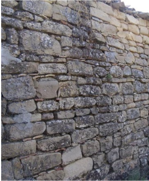
Fig. 4. Detail of a wall in Porcuna without mortar ( a hueso construction). (Source: Belmondo, Millán, 2022).
