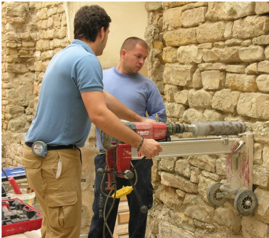
Fig. 7. Detail of the process of extracting the stone from a load-bearing wall to analyse its internal composition. It is possible to observe that the wall is without mortar but just a mud poor in lime. (Source: Millán, 2014).
