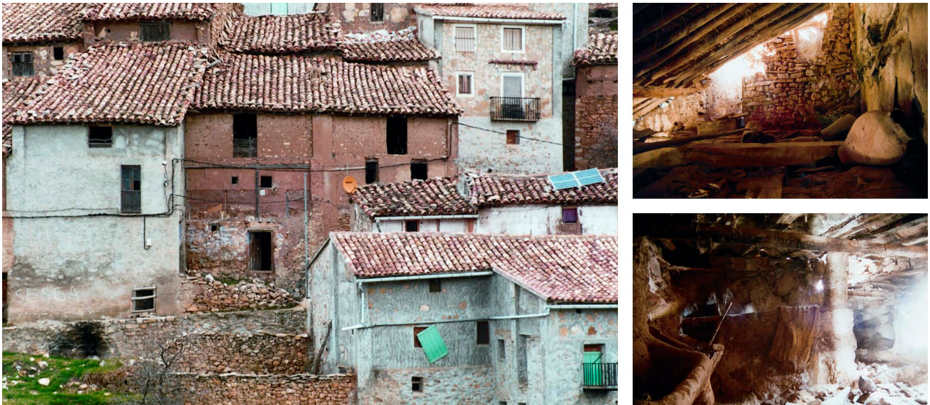
Figure 3. The house before the intervention. Credits: C.M., F.V.
