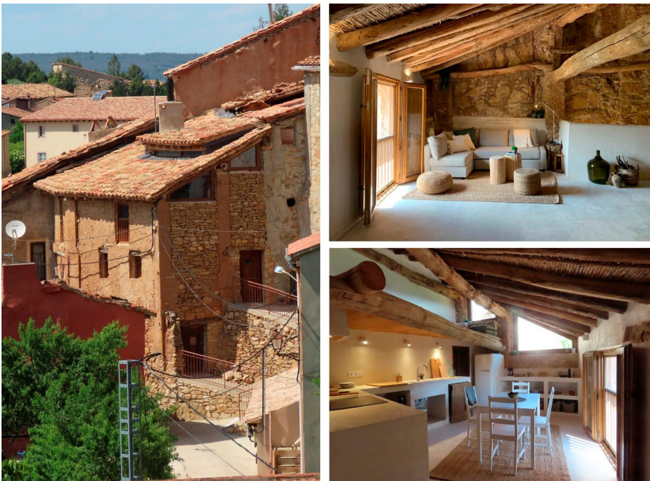
Figure 4. State of the house after refurbishment of its external facades and internal spaces. Credits: C.M., F.V.
