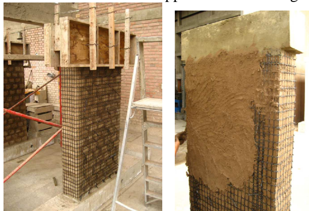
Figure 1. Building of the tested walls
