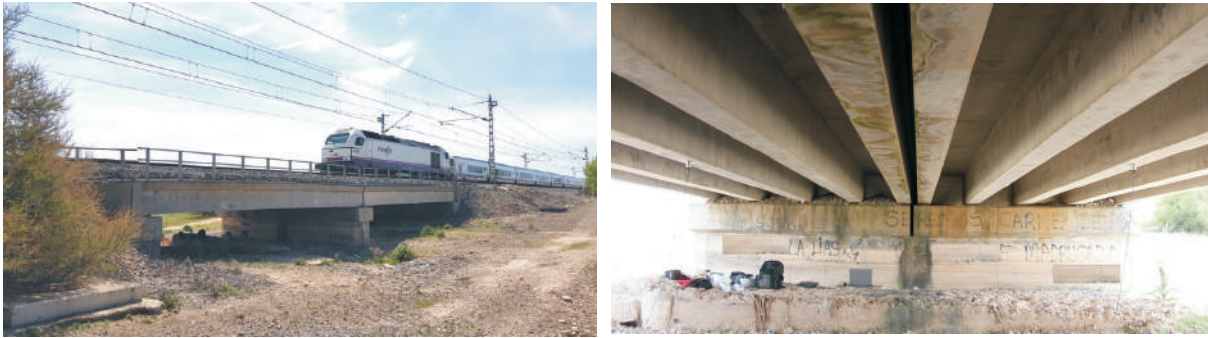
Figure 12. Old Guadiana River Bridge.
