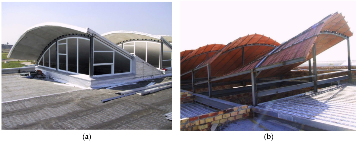
Figure 6. Views of the new skylights. (a) Final view; (b) under construction.
