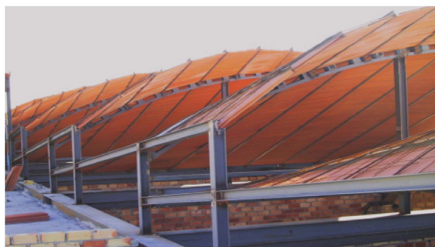
Figure 7. A view of the new ceramic vaults.
