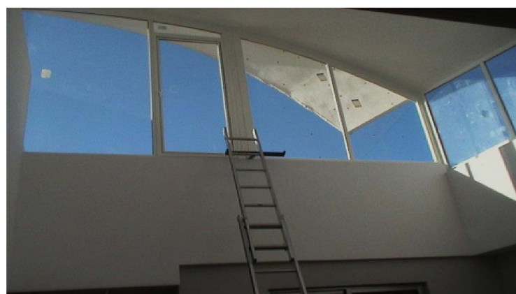
Figure 8. The interior view of the aspect of the residential units with vents for aperture.
