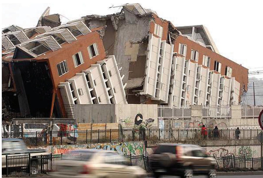
Figure 5. Alto Rio Building, after the 8.8 Mw earthquake in the city of Concepción. Source: emol.cl.
