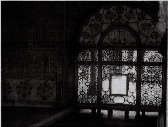
Figure 2: An exquisite jalis at Lal Qila (Red Fort) New Delhi (India). Notice also how if necessary, water can be conducted under the screen to further enhance evaporation.
