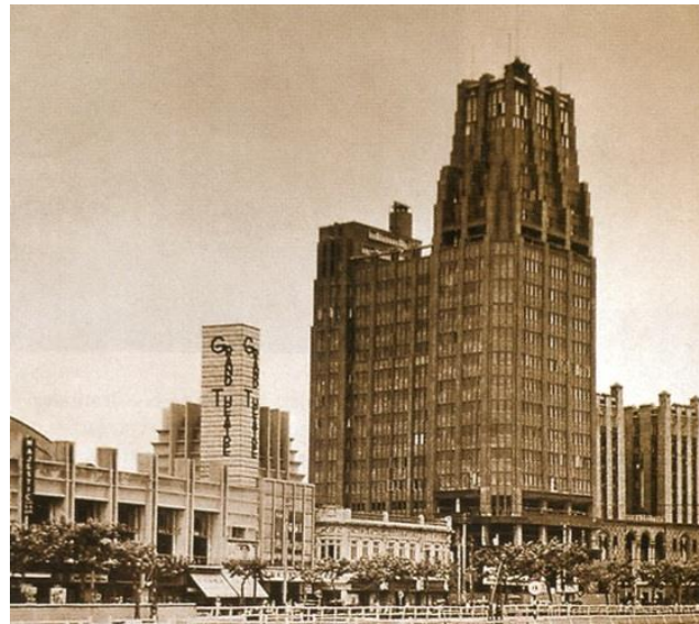
Figure 15. View from the racecourse towards the Grand Theatre and Park Hotel.
