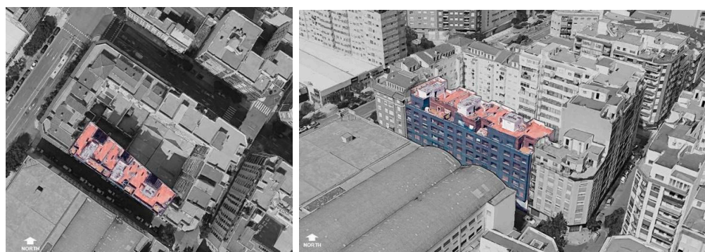
Figure 3. Panoramic view of the building—Main façade is oriented to the southwest according to urban plot. Source: [31].
