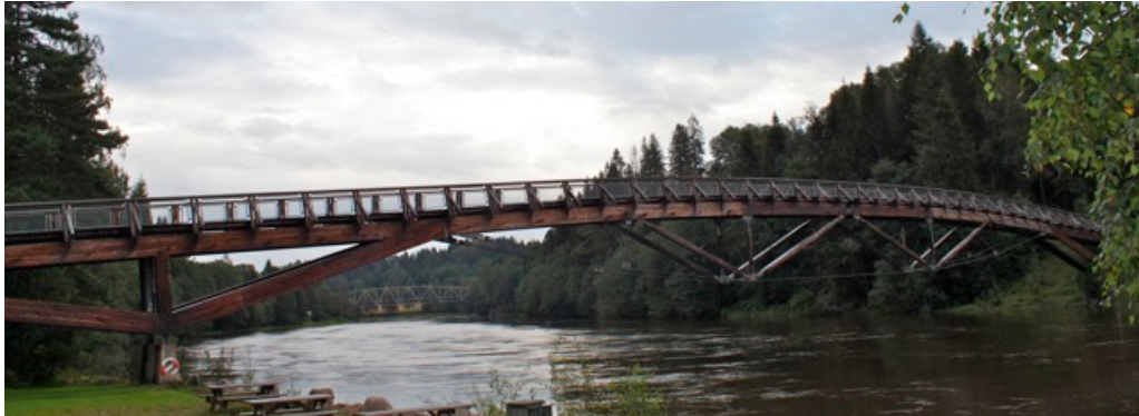
Figure 9. The Lardal footbridge. (Picture after http://broer-vestfold.blogspot.com/2011/08/bro-v-kjrra-fossepark-i-lardal.html ).
