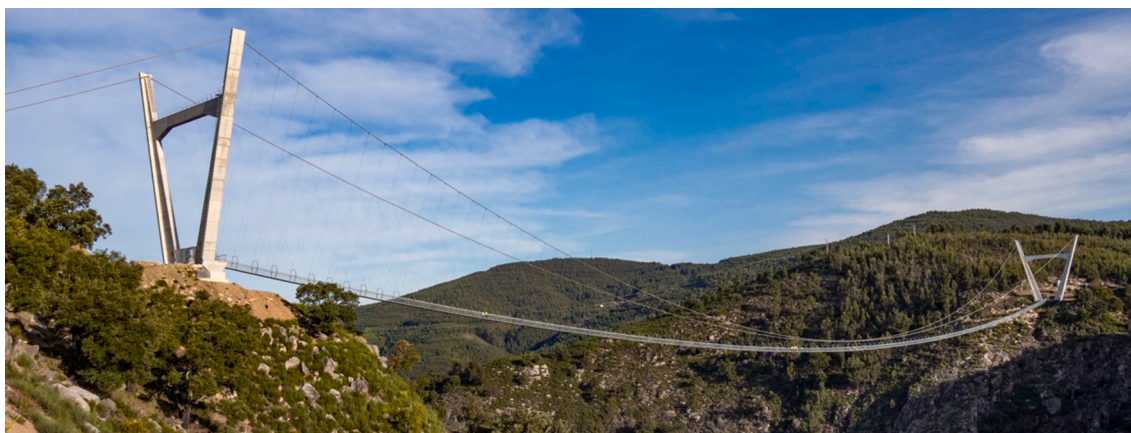
Fig. 1. View of the 516 Arouca footbridge (Portugal).
