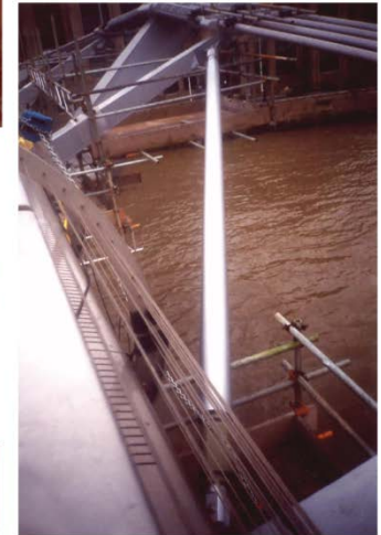
FIGURE 8 PIER DAMPERS
