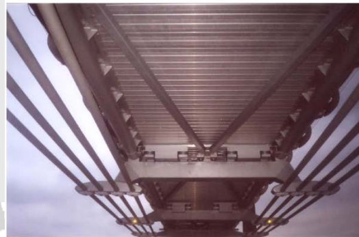
FIGURE 9 CHEVRON DAMPER
