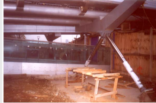
FIGURE 7 VERTICAL DAMPERS
