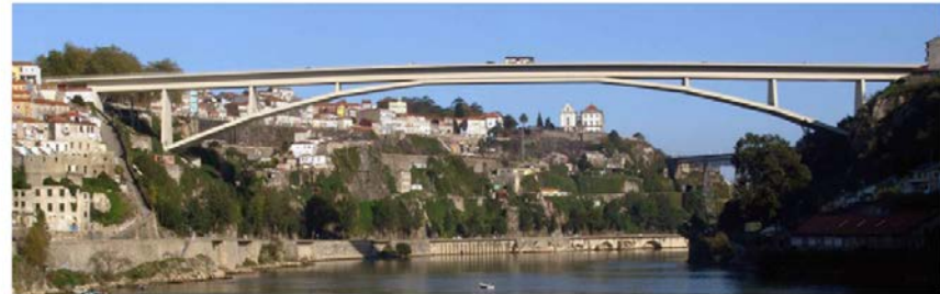
Fig. 1. View of Infante D. Henrique Bridge from downstream (Porto at the left side).
