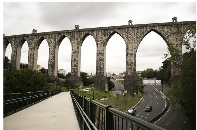
Fig. 9 Lisbon, Vale de Alcântara pedestrian bridge. Source: the authors, 2020.
