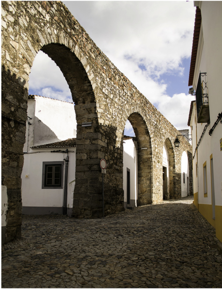
Fig. 5 Évora, Água de Prata Aqueduct's urban stretch. Source: the authors, 2020.
