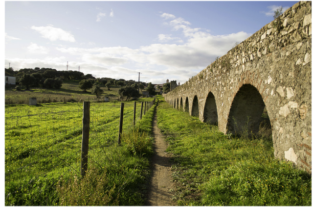
Fig. 6 Évora, Água de Prata Aqueduct's rural stretch. Source: the authors, 2020.
