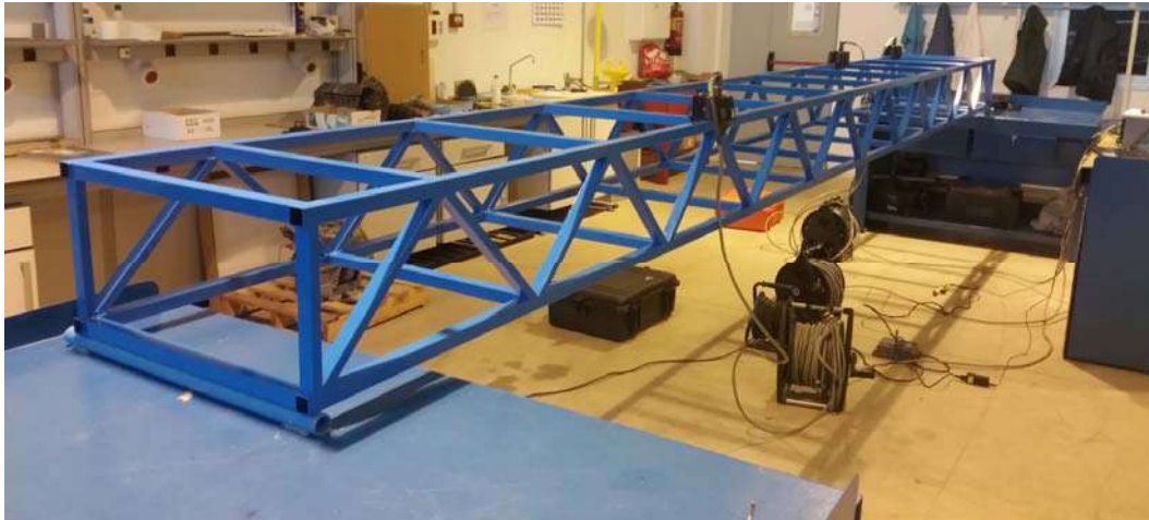
Figure 2. Laboratory footbridge at the Universidad de Almeria.
