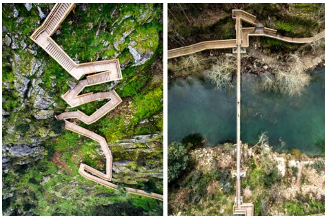
Figure 9. Trimétrica, Paiva River, (Arouca, Portugal), 2015. (Source: Image courtesy of Nelson Garrido).
